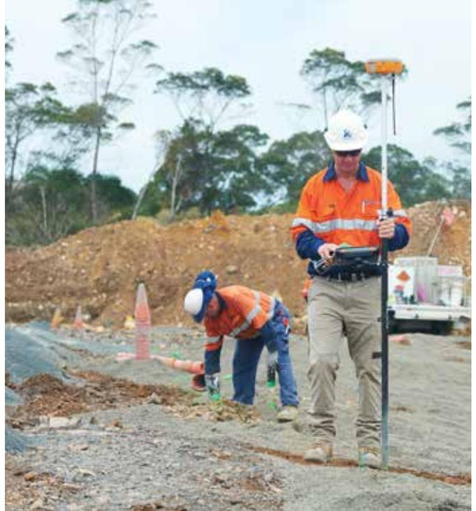
Orica blast surveyor Cameron Ingles uses the GPS Rover on a bench at Boral Dunmore.
