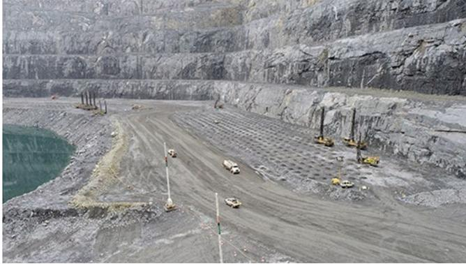
Figure 3 - Part B, drilling adjacent to MSF temporary haul road
