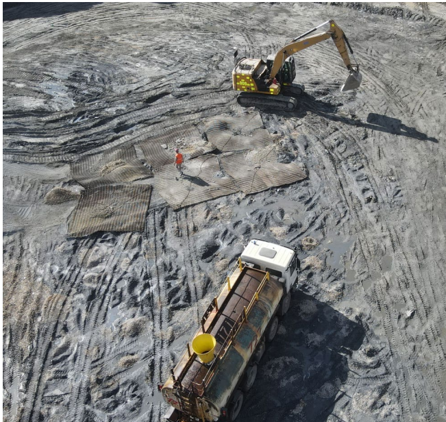
Figure 8– Watering and placing blankets on a WebGen™ blast.
