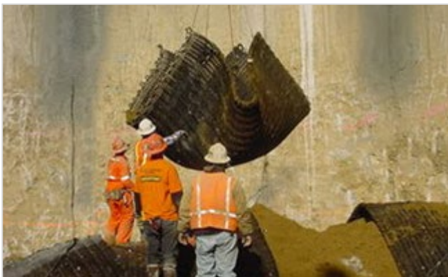
Figure 3 – Using mats on the blast to control rock ejection.
