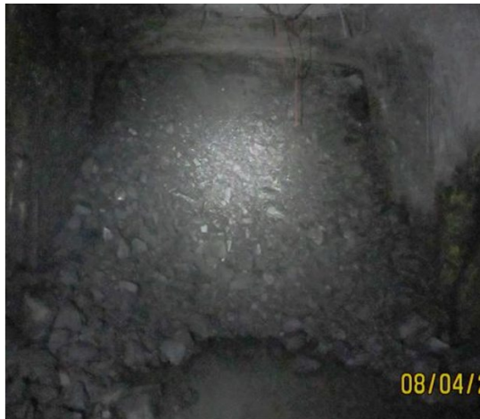
Resulting blasted stope
