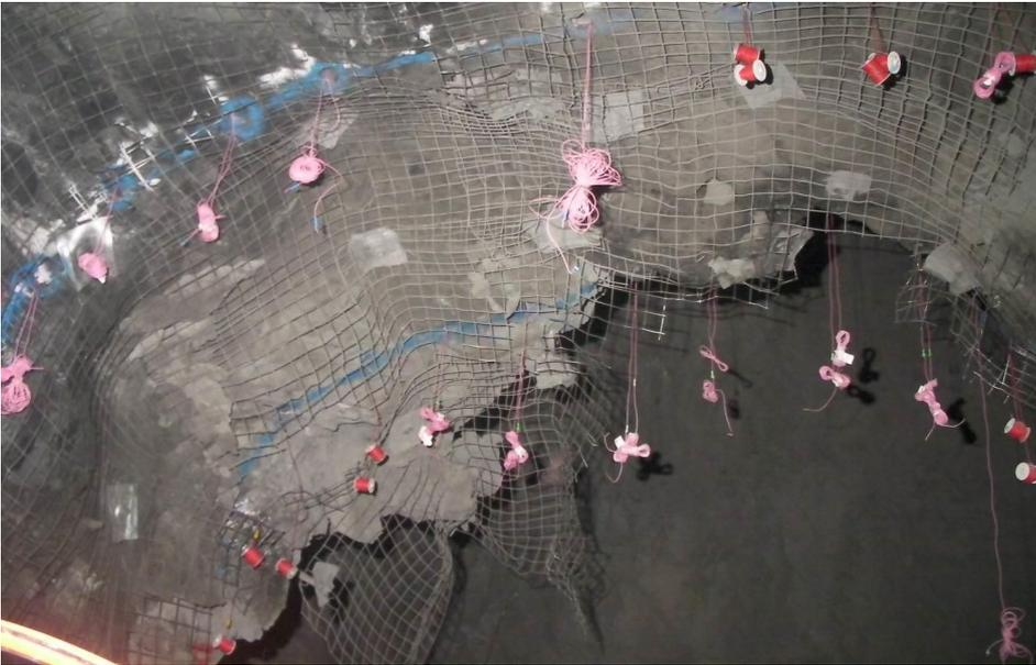
Figure 7. Charging complete for the Hook-up process to tie it into the detonating cord at the open stope brow
