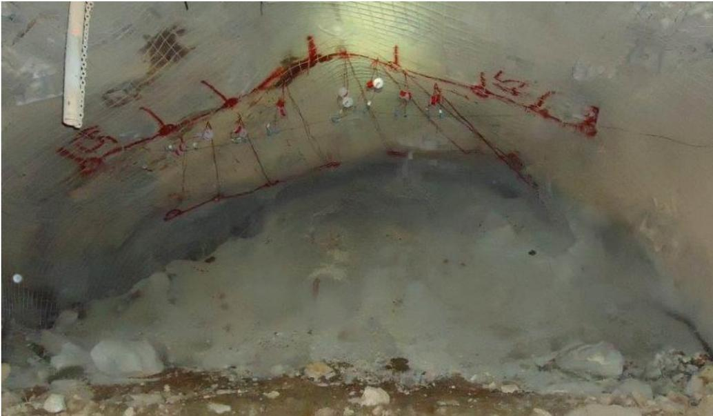
Figure 5 Hook-up for a single SLC ring with risks partially controlled with backfill, shotcrete and bunding
