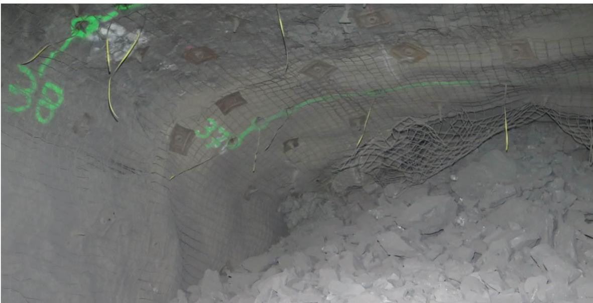
Figure 6 2 Multiple wireless charged rings are ready to fire as soon as needed, note strapping indicators.
