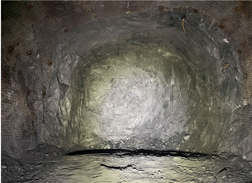
First Avatel™ blast after mucking
