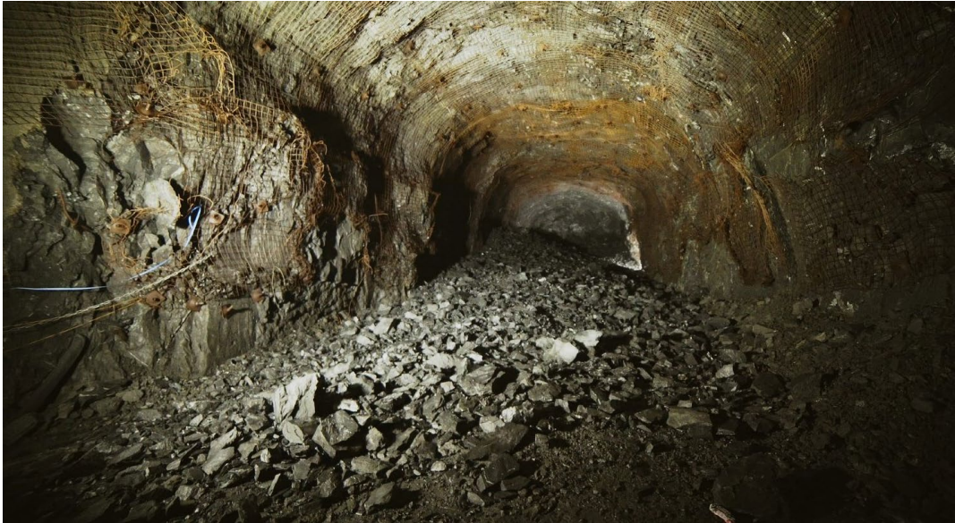
The blasted face charged by Avatel™
