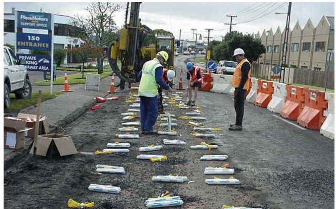
Figure 1: i-kon™ trench at Marua Road, Auckland.
