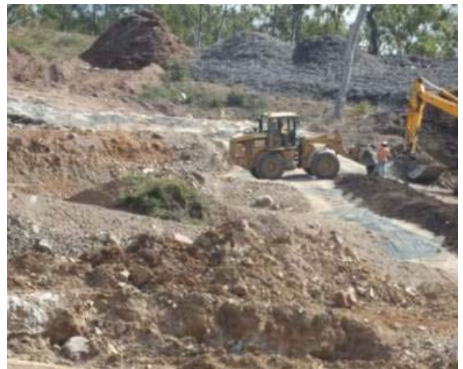
Covering of the trench blast to assist in flyrock control
