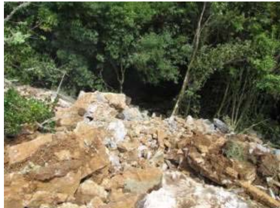
Minimal Material in Creek
