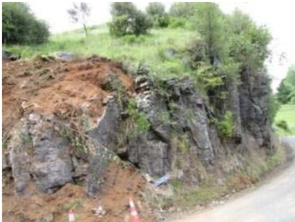
Limestone face to be removed – looking south west
