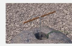
**1.9** Lower the charge using the rope. Touch hole bottom. Suspend the charge using the dowel and rope. Ensure rope takes weight and not detonating cord.
