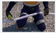
**1.4** Cut off excess cartridges.
