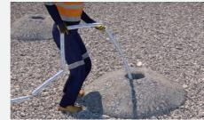
**1.3** Lower cartridges to the bottom of the hole. Pull up the length equivalent to uncharged collar length.
