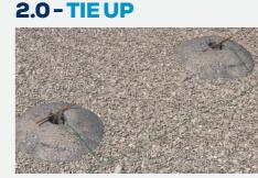
**2.1** Layout trunkline. Based on this product's compatibility tables, Cordtex<sup>™</sup> 10 or 10P (as a receptor) is compatible with a 5gm cord.
