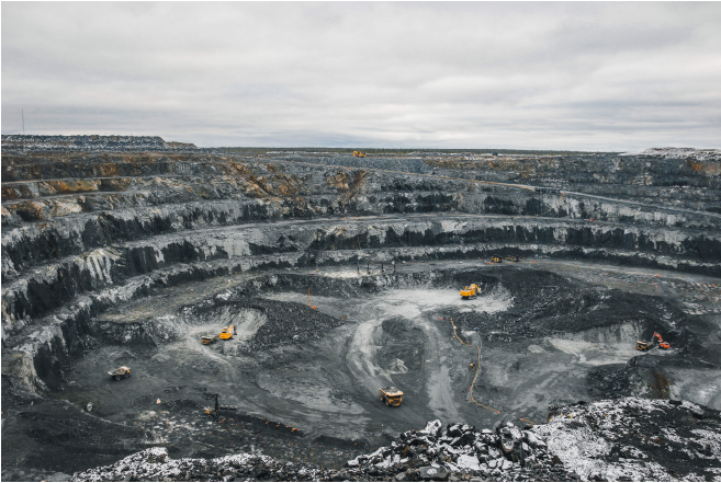
Figure 1 – Kevitsa site overview
