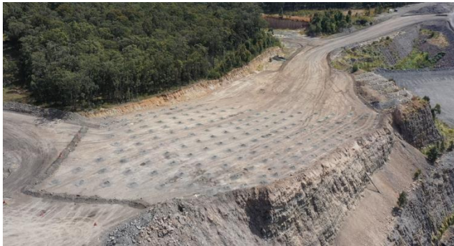
Blast pattern EX05_B1_S1 just below the pre-strip zone.
