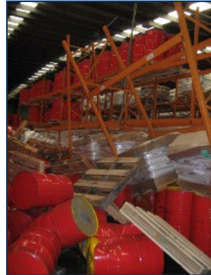
The Chemicals warehouse sustained damage to pallet racking which had to be methodically cleared.
