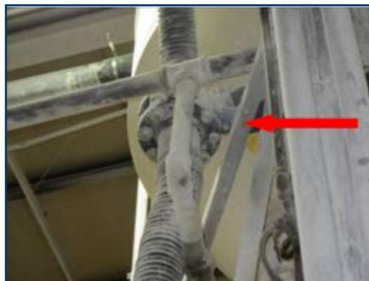
The knife valve was installed in the mixer exhaust lines.
