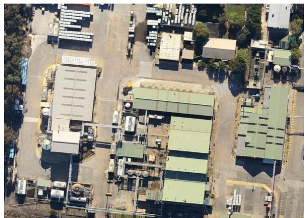
Orica Deer Park Emulsifier Plant – Melbourne, Australia
